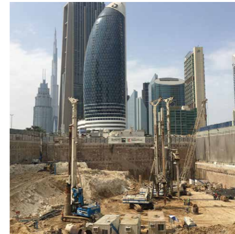
ICD Tower foundations - Dubai
