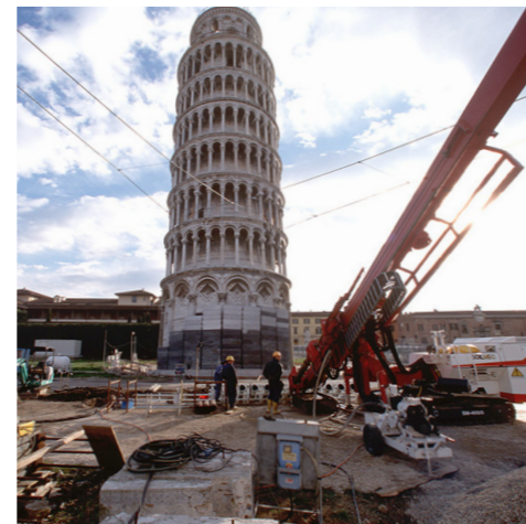
Tower of Pisa foundation remediation - Italy
