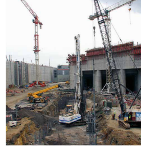
Doubling of the Panama Canal - Panama
