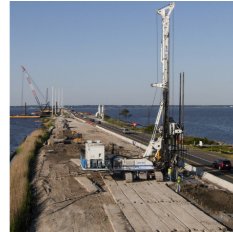
US 331 highway, Florida - USA
