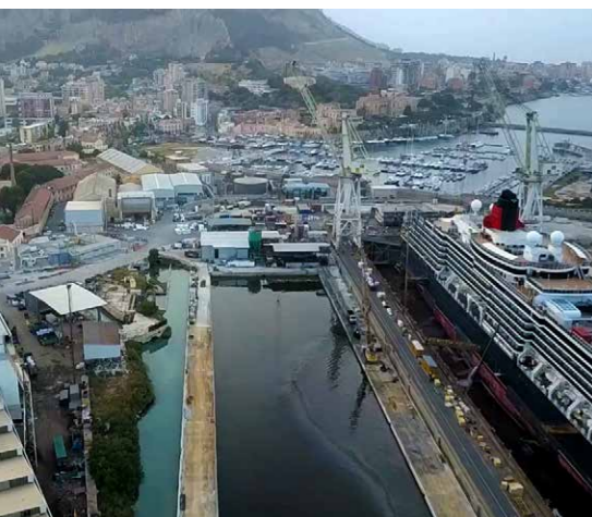
Environmental recovery, dry dock, Palermo - Italy
