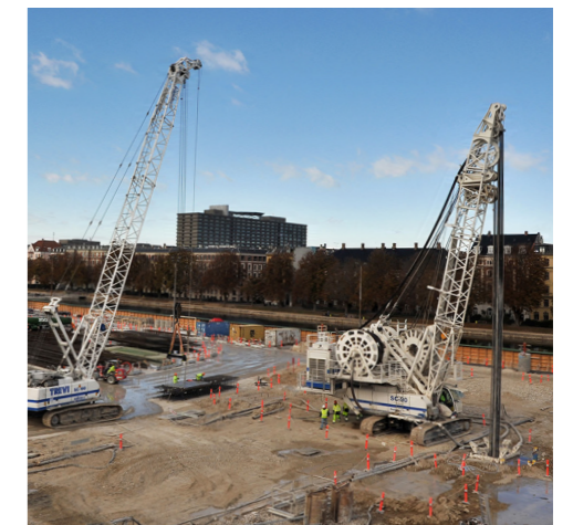
Copenhagen underground foundations - Denmark
